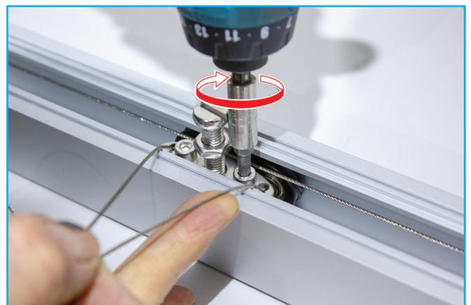
**5.** Slide the A hanger into the stop (96200-1) while holding onto the cable. Tighten the hexagon screws of the A hanger.
